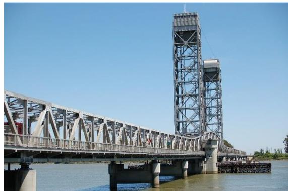
The project will preserve the Rio Vista Bridge over the Sacramento River by cleaning the surface, removing the old paint and then repainting all steel surfaces. The work is expected to take two to three years to complete.
